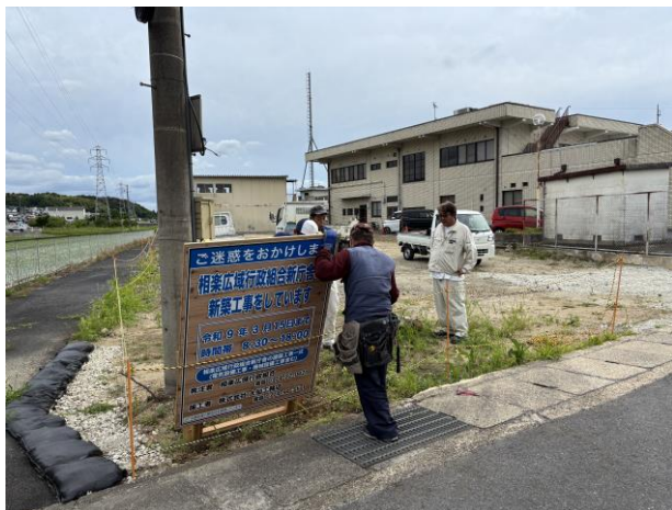
▶工事看板設置中(R8. 6. 23)
