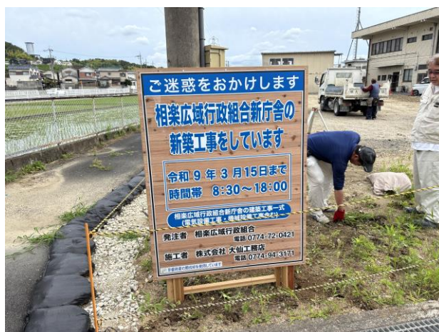
▶工事看板設置完了(R8. 6. 23)
