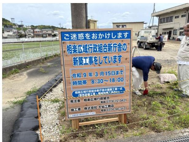
▶工事看板設置完了(R8. 6. 23)
