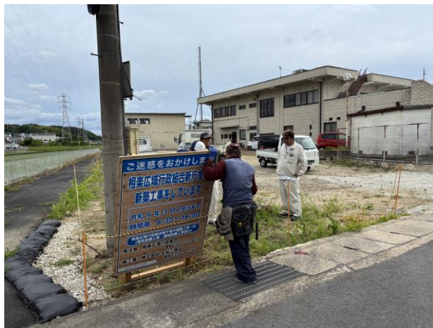
▶工事看板設置中(R8. 6. 23)
