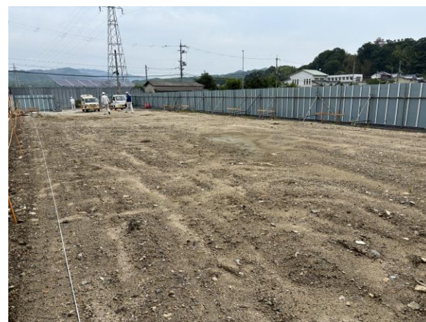
▶仮囲い完成(R8. 6. 30)
