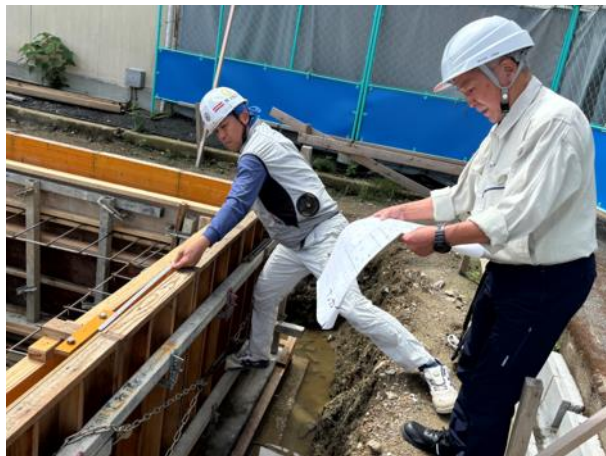
▶アンカー検査(R8. 9. 10)
